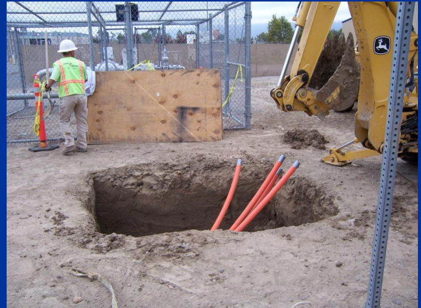
Directional Boring of Underground Conduits
