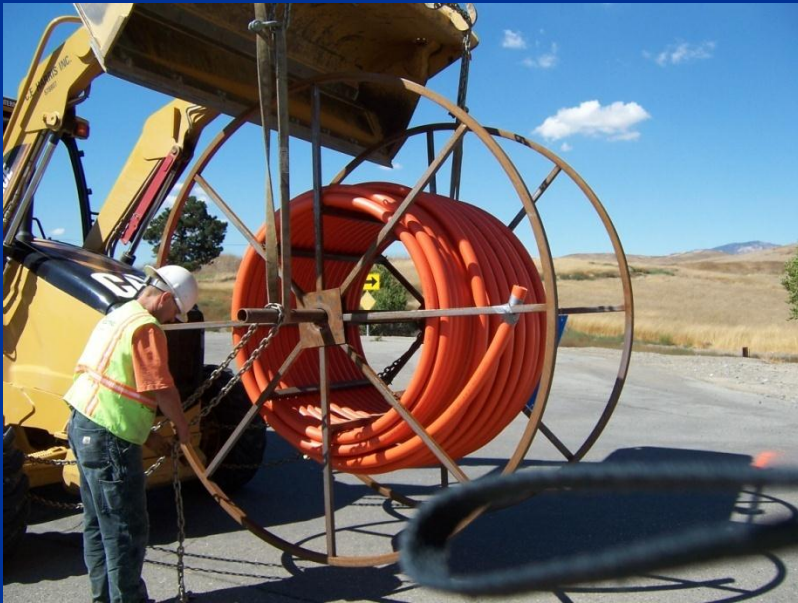
Directional Boring of Underground Conduits
