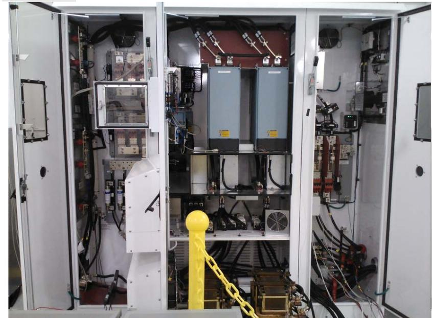
*The schematic and a picture of the 500kW grid connected voltage source inverter.*
