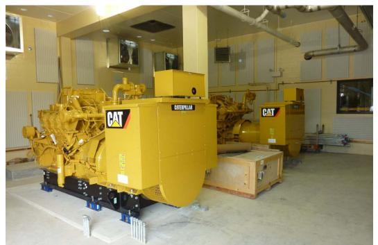
Figure 10 - Engine generator sets at Beaver Dam. Photo courtesy of Wayne Karlovich, Applied Technologies, Inc.
