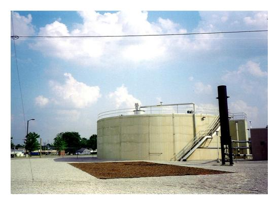
Figure 13 - General Mills Complete Mix Tank Digester. Photo courtesy of Dennis Totzke of ATI.
